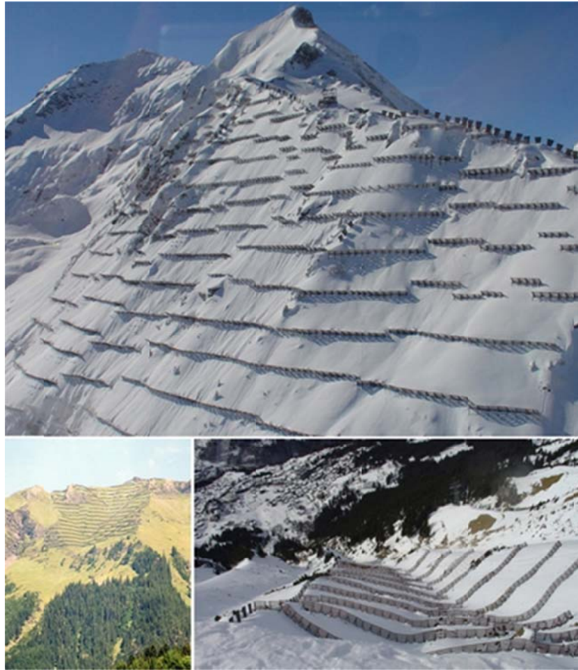
Figure 1: Photograph of snow supporting structures typical of European deployments.
